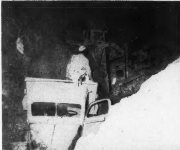
LEFT: Leonard Steen, operating the Caterpillar D-2 with Traxcavator loader, trips a skip-load of ore into the Chevrolet truck driven by John Sluka. Because the scheelite-tactite ore is unusually heavy, Leonard handles less than a full scoop of ore each time. RIGHT: Standing on the ground, Al Lambert talks to Earl Dye, a young friend who is sitting in the seat of the Caterpillar D-8 that is used for exploration, prospecting, and some pit work. The ripper has allowance for five teeth, but is fitted with only three teeth so that it will dig better in unblasted rock.
